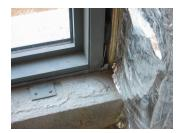
This photo shows a curtainwall sill corner in a building under construction, in which we can see sill fastener clips that penetrate the sill flashing, backer rod braided like a rope, and flashing corner
