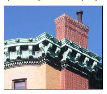
We examined the copper cornices and were able to reattach pieces that had come loose, avoiding an expensive replacement program. Chimneys were completely rebuilt.
