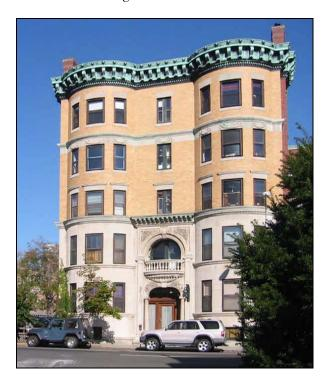
Exterior masonry on the Brentford Condominium was restored over a period of several years, with the most critical areas addressed first. Areas that were re-pointed blend visually with the areas that were not repointed, avoiding the need for a total repointing.
