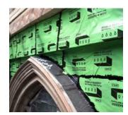
Granite facing was reinstalled over a new membrane and copper flashings.
