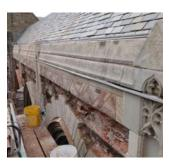
First we addressed severe rusting in a beam that was cracking the masonry
