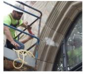
Pumping air into the joint makes a puff that shows a void extends through the arch.
