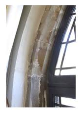
Chronic water damage came from water seeping through joints in the arches, even after the masonry had been re-built with a water barrier under the veneer, and new flashings over the arches. We knew from experience that the mortar joints in arches usually have gaps in the mortar. It is very hard to pack these sloped joints full when setting the massive stones of the
