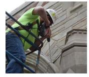
Drilling through the mortar joint to inject flowable grout
