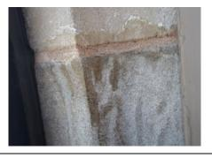
Water seeping straight through mortar joints, even after installing the flashings and water barriers.
